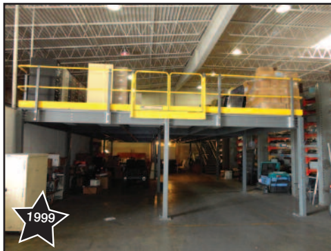
Wildeck 27'x60" Steel Mezzanine
