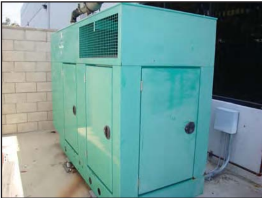
Onan Cummins Quiet Site 100KVA Diesel Generator w/Power Command Transfer Switch.
