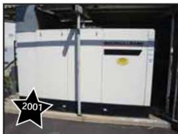
(2) IR 125hp Rotary Air Compressors
