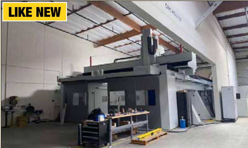
CMS Poseidon 50/130 KX5 Z2500 NC, Boring-Routing-Milling Machine Room
