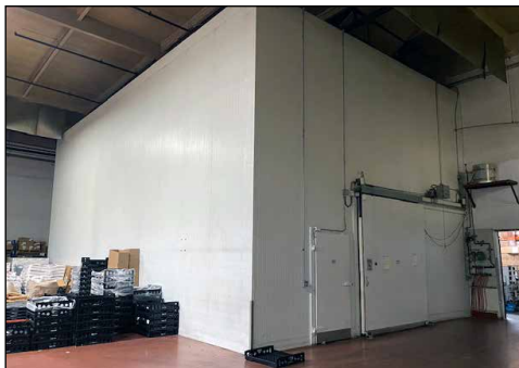
R' Cold 30' x 20' Cooler Room
