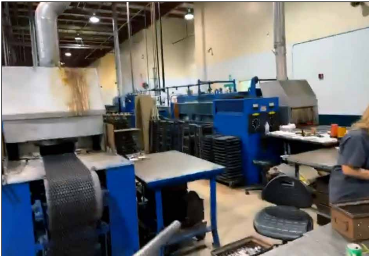
Lindberg 17-SC-20810-21A24C Exothermic Furnace
