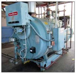
Cleaver-Brooks Mod. CBH-799-50 CBM Packaged Boiler
