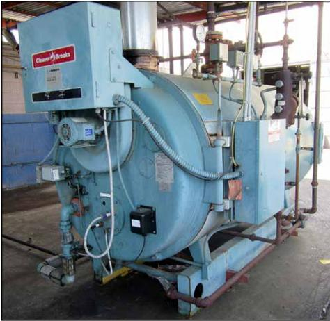
Cleaver-Brooks Mod. CBH-799-50 CBM Packaged Boiler
