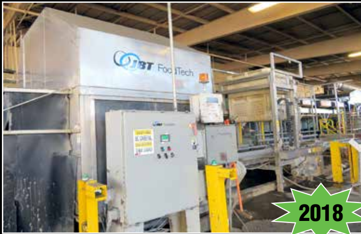
MAF Bin Wash Line
