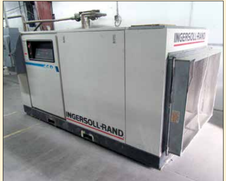
Ingersoll-Rand 75hp, SSR Mdl. SSR-XF75 Air Compressor
