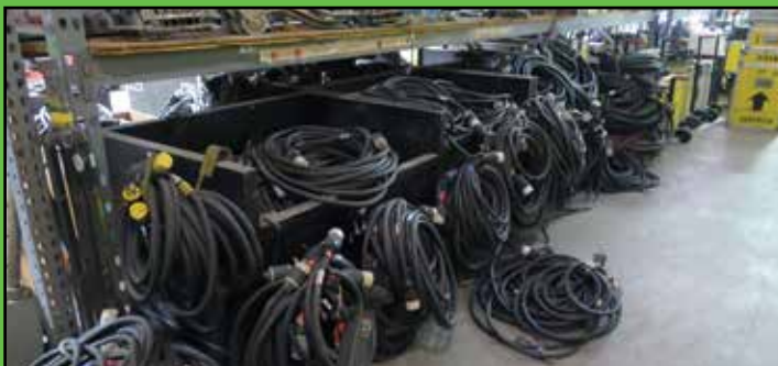
View of Cables
