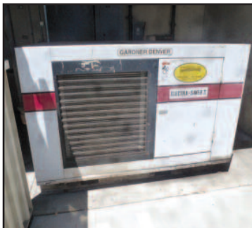
Garner-Denver Electra Saver II Air Compressor
