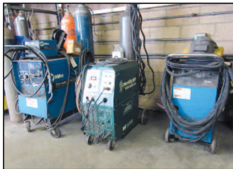
Partial View of Welders
