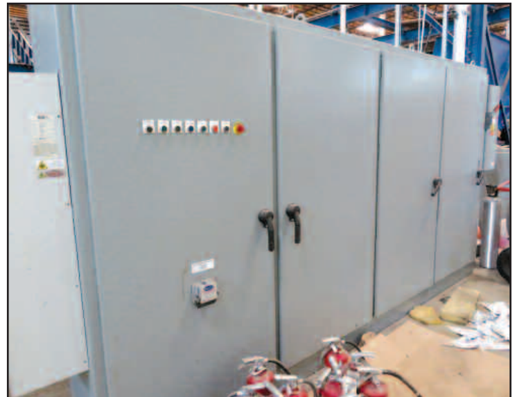
Shredder Motor Control Center
