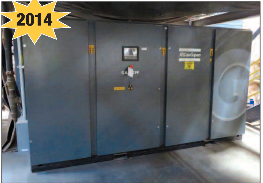
Atlas Copco 189HP Rotary Screw Air Compressor
