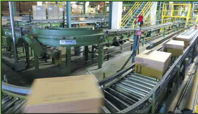
Bushman Power Inventory Transfer Conveyor
