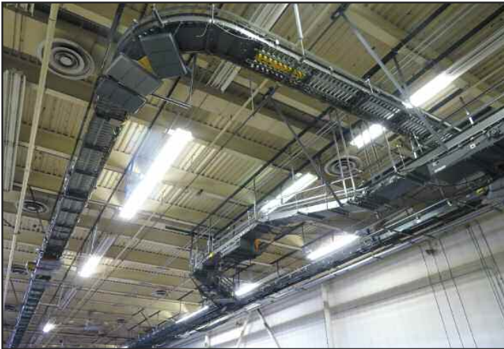
18,000 Linear Feet Bushman & FKI 18”-22” Power Roller & Belt Conveyor
