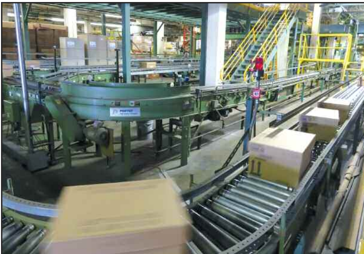
Bushman Power Inventory Transfer Conveyor
