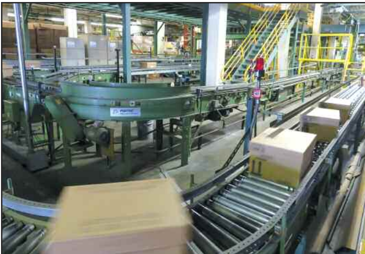
Bushman Power Inventory Transfer Conveyor
