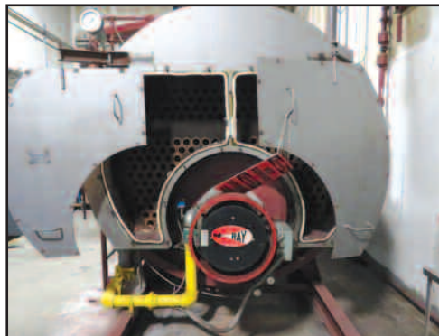
Johnston 300hp Boiler
