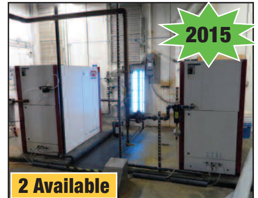
Gardner Denver 37KW Compressors
