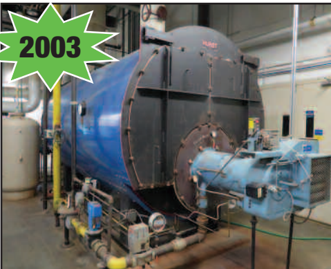
Hurst 16MM BTU Boiler
