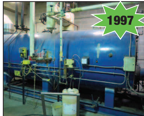
Hurst 150 PSI Boiler
