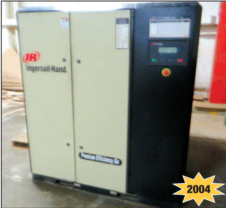
I.R. 60 H.P. Rotary Screw Air Compressor
