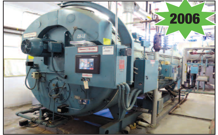
Cleaver Brooks CBI-700-350-150 Boiler
