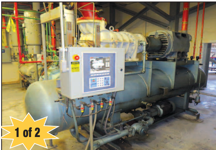
Mycom 500 hp Refrigeration Compressors
