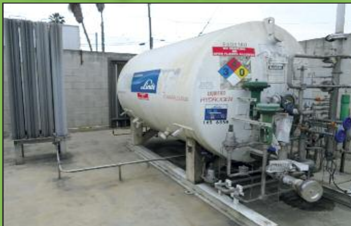
Linde 1500 Ga. Cryogenic Tank
