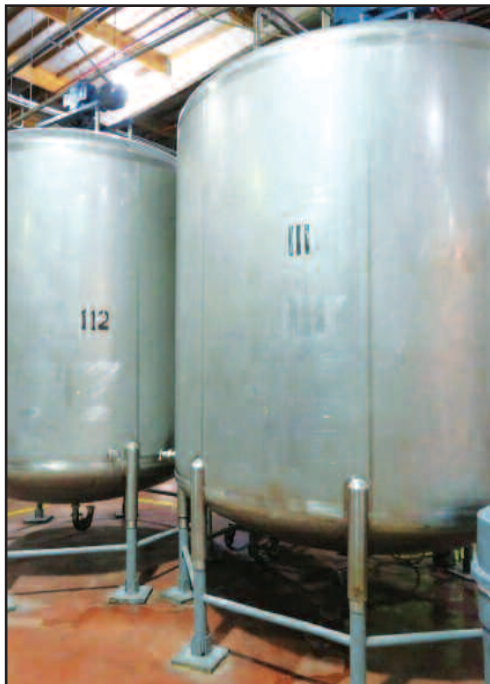
5000 Gal. 316 S.S. Holding Tanks
