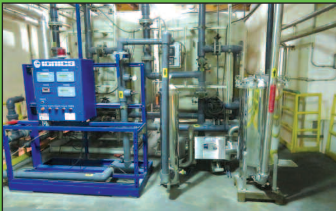
G.E. Ionics U.S.P. Water Purification System
