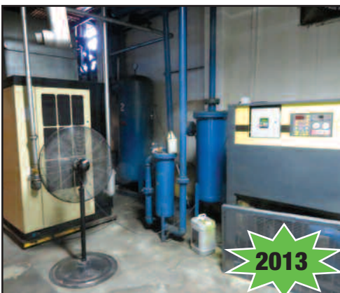
I.R. 150hp Rotary Screw Air Compressor
