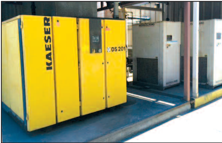
Partial View of Air Compressor Department
