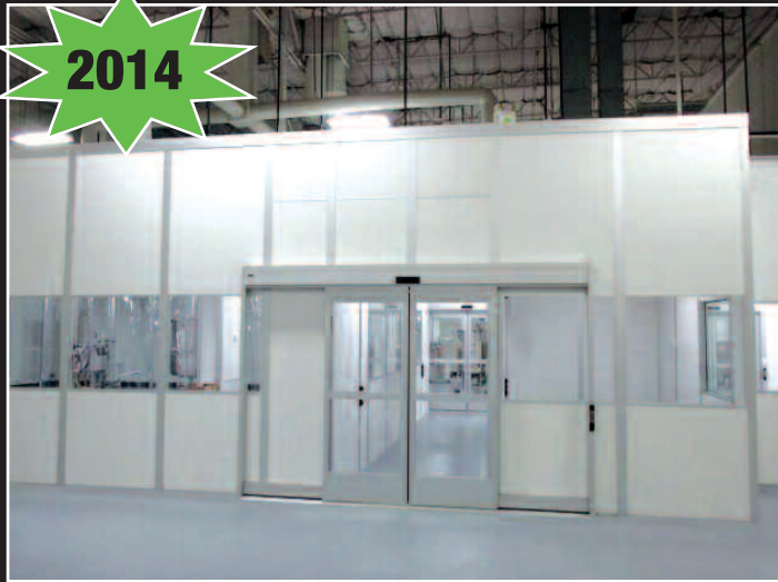
ACS 4000 Sq. Ft. Modular Clean Room
