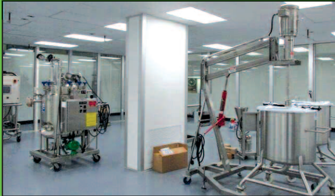
Overall View of Clean & Process Room
