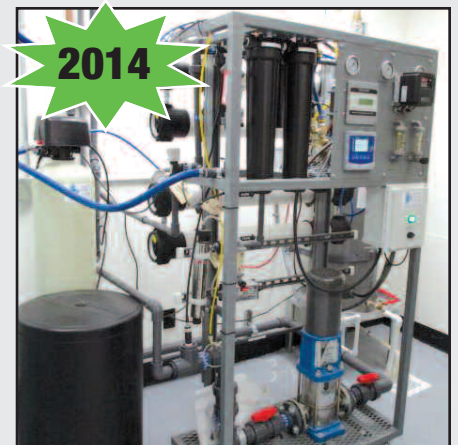
So. Coast Reverse Osmosis System
