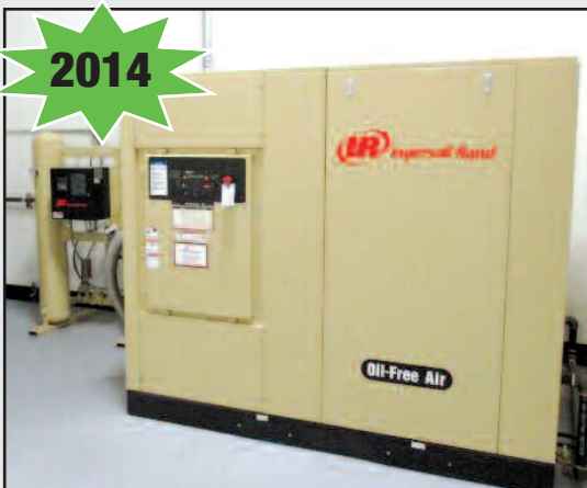
I.R. 50hp Rotary Screw Air Compressor
