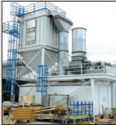
Donaldson/Torit 100hp Cyclone Dust Collection System
