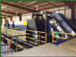
View of Recycling Line
