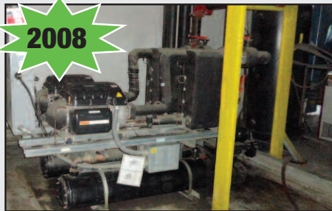
Thermal Care TCW 140 Ton Chiller
