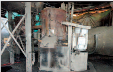
(2) 200hp Belt Drive Densifiers
