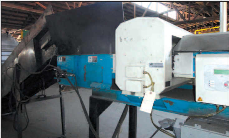
Pelletizing Line / Feed System
